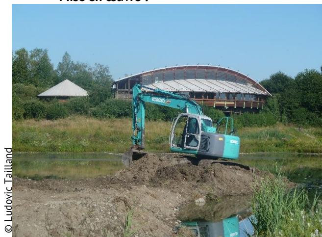
Figure 1. Intervention de curage
